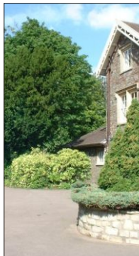
Conservation: The Beeches Hotel, Bristol
