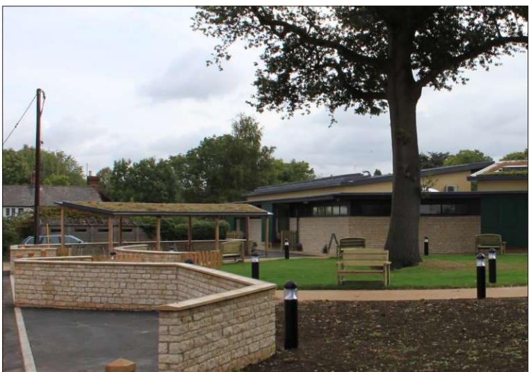
School at completion. September 2011
